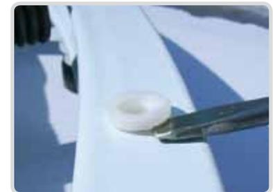
**Trimilin-sport:** Check the protective eyelets in the frame regularly! If there is a pronounced notch you can lift the eyelet and turn it around. First lift it with a screwdriver. Then turn it 180 degrees around and push it back into the frame.
